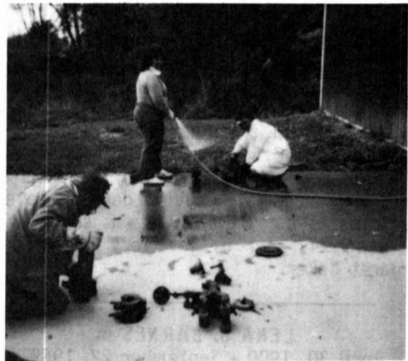
Judy hoses off acid, as Doyle and J.D. use wire brushes to remove excess rust.
