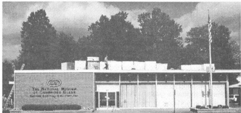
The materials for the new roof, ready to go.
